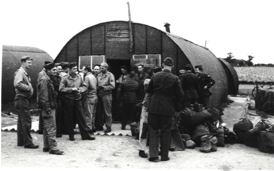
Going Home – 325 th SCS men look on, as some 'Happy Warriors' wait for the truck to take them to Royston Railway Station to begin the long journey home.
